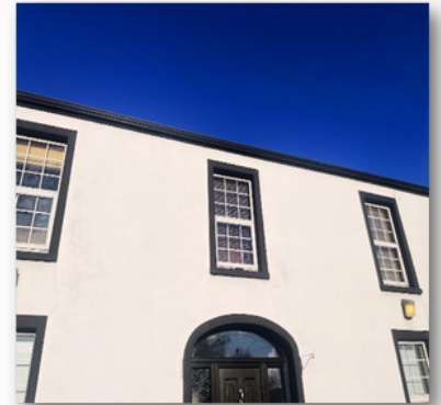
Front door of The Beeches RC photographed by Alastair McShane
